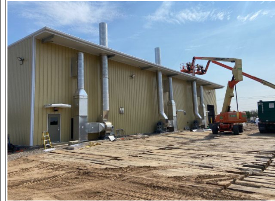
Photo Caption: Installing Fan Duct/ Installing Supports
